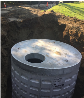
Dry Well Installation
